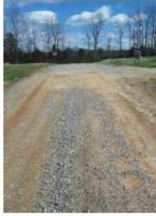
End of unpaved section of road. Remaining 150' to the intersection will receive tar and gravel as well, to ensure uniformity once the unpaved portion is complete and surface treated.
