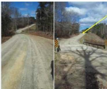
Existing rock riding surface in this hill. This stone will have to be blasted and removed during construction.
